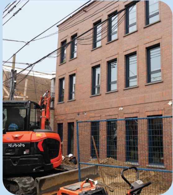
Monk Pavilion construction site
